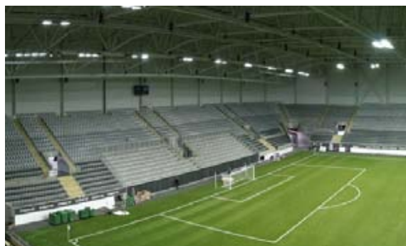
INDOOR STADIUM TALLIN - (ESTONIA)
